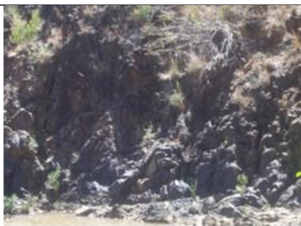
Plate 2.3: Highly weathered Samburu basalts upstream of the bridge site
