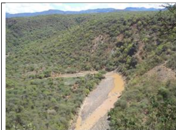
Plate 2.1: The Radat dam site and catchment area, note sediment deposits on the river bed and high water turbidity due to catchment degradation.
