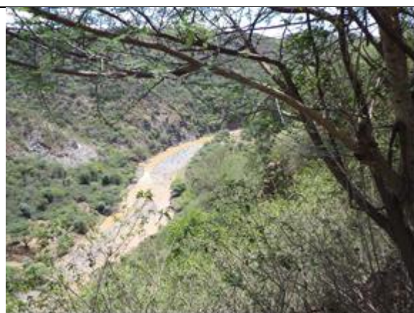
Plate 2.2: The Kopokaplelach dam site on Kapuchara river
