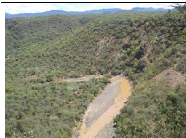
Plate 4.1: The Radat dam site and catchment area, note sediment deposits on the river bed and high water turbidity due to catchment degradation.
